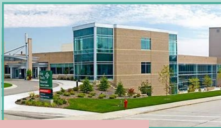
Present Front Entrance
